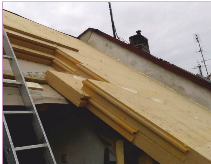
Isolair 2 x 120 mm = 240 mm
